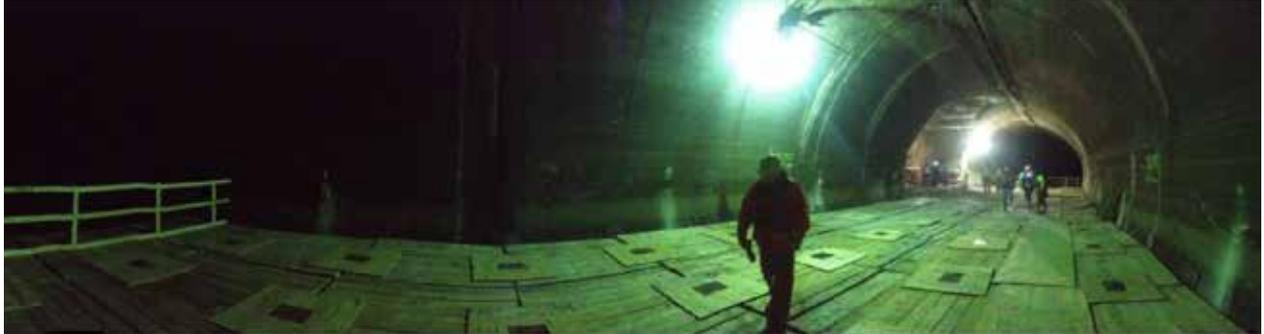
Tunnel with a pilot tunnel. A ramp was constructed on the dry side of the pilot tunnel using the shot rock. Later, the pilot tunnel opening was enlarged with additional rounds of blasting and jack hammers. The ramp was kept at a higher elevation than Mainstream Tunnel invert to allow installation of a temporary work platform (access deck) using timber decking mats over the water in tunnel. Once initial steel set beams (W14 x 109) were anchored in
