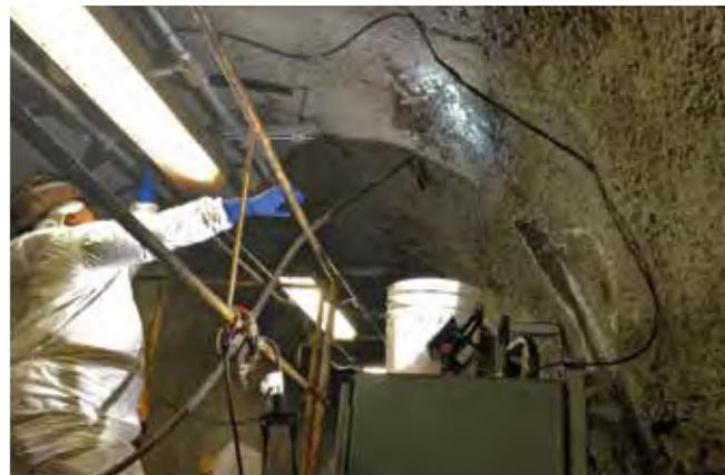
Chemical grouting to prevent water inflow into a subway tunnel.
