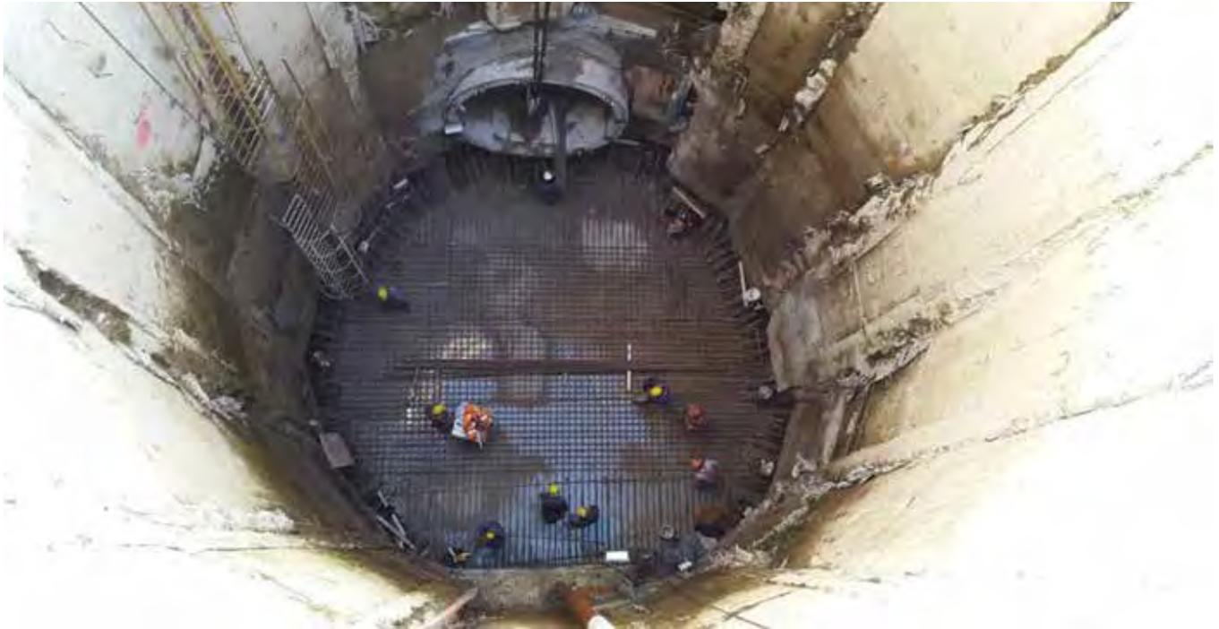
closure. For confirmation, the shaft was evacuated in a controlled pump-down test over a period of four days. The water level of the shaft was continuously monitored and compared against the piezometer levels. This ensured that there was no communication between
