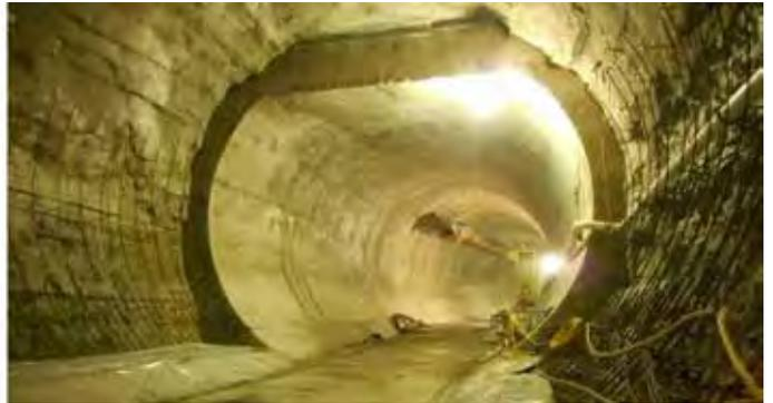
The existing nominal 305-mm (12-in.) thick unreinforced concrete liner was scribed with a radial saw cut at the limits of replacement that are established by the structural engineer's inspections and evaluation of field and lab test results.
