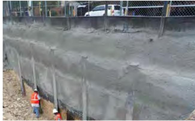
Temporary soldier piles and lagging for earth retention to facilitate tunnel construction.
